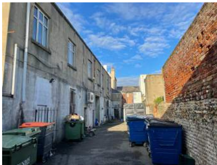
2. Exterior, service yard
